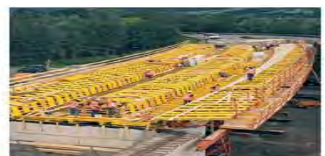
A cost-effective solution: Bridge formwork with GT 24 girders.
