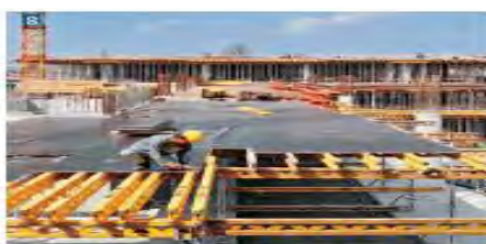
The GT 24 as formwork girder with MULTIFLEX slab formwork.
